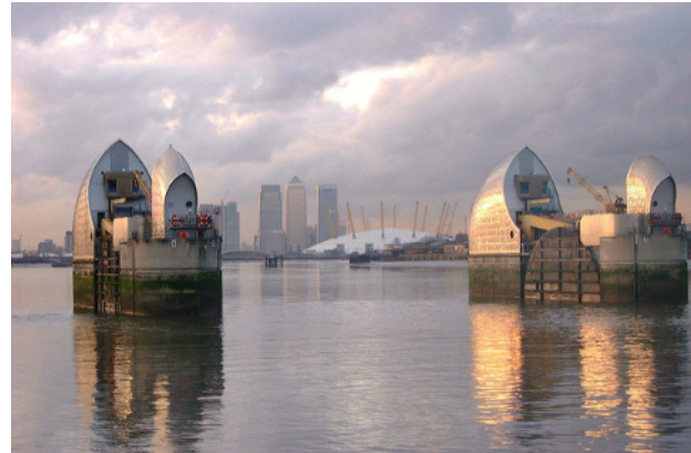
Figure 21. The Thames Barrier. © Ken Brown.
