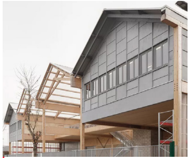
The Cycle Terre factory, created as a cooperative by several companies and territorial authorities, transforms the raw earth of rubble from building sites in Ile-de-France into construction material.
